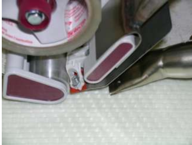
Figure 6: Application of the adhesive-primer using a heat source and a small roller.
