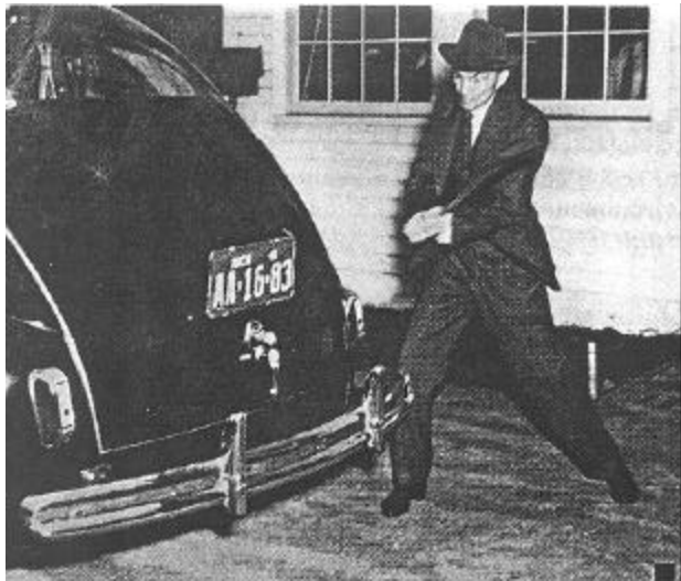
Figure 3: Soy protein plastic based composites (Henry Ford 1941)
